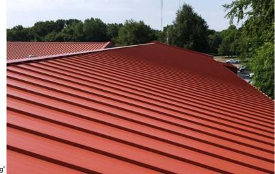
Oil canning: Union Corrugating Company purchases prime commercial grade light gauge metal which is manufactured to all industry accepted tolerances. "Oil canning" is an inherent part of light gauge cold formed panels and is not cause for rejection.
